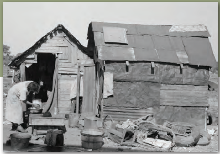
During the Great Depression, loss of jobs and farms forced many to relocate. Shanty towns, known as "Hoovervilles," cropped up across the country, often located in or near the city dump. This family home at the Oklahoma City dump (South May Avenue) was photographed by Russell Lee, July 1939, documenting what he identified as "May's Avenue Camp." Library of Congress
